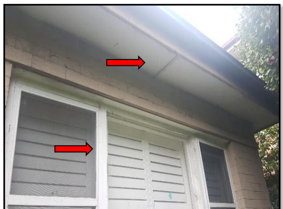
Photo 12: Image of potential lead paint and suspected ACM eaves at 9 Fig Tree Street.
