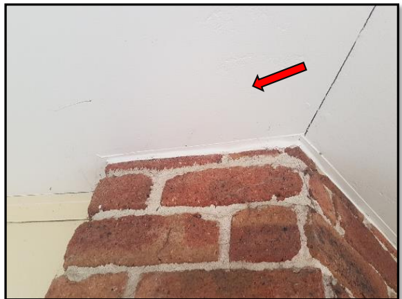
Photo 16: Image of potential ACM eaves observed at 15 Fig Tree Street, near BH05.
