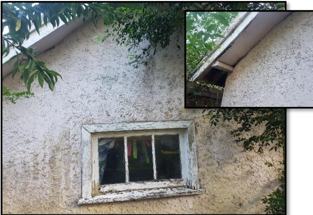
Photo 3: Image of additional structure observed at 106 Centennial Ave, with possible lead paint on window frame and (insert) suspected ACM eaves.
