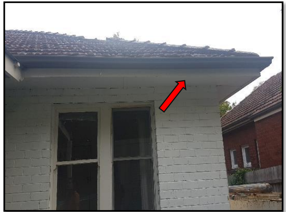
Photo 8: Image of house at 110 Centennial Ave, with suspected ACM eaves.
