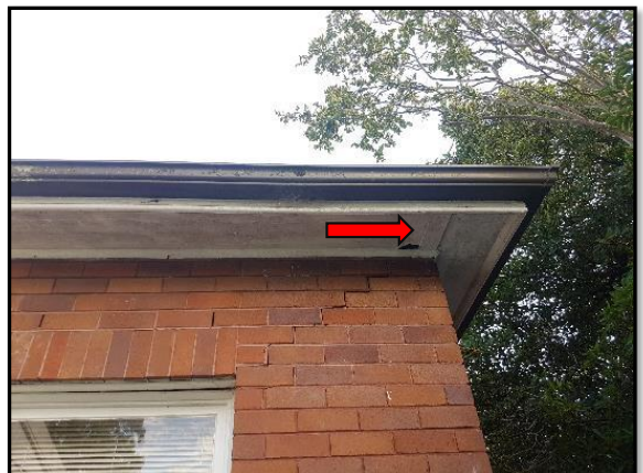
Photo 6: Image of suspected ACM eaves at 108 Centennial Ave on house.
