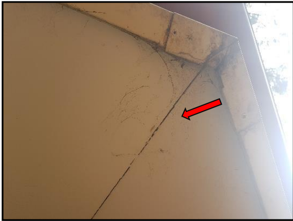
Photo 15: Image of suspected ACM eaves observed at 15 Fig Tree Street, near BH05.
